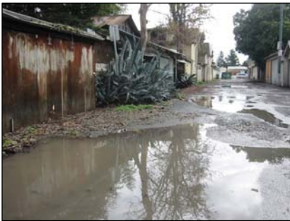
Two alleyways in poor condition in the Spartan Keyes SNI Area.
