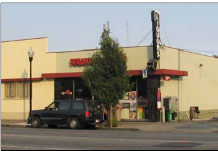
Stadium Liquors after façade improvements.
