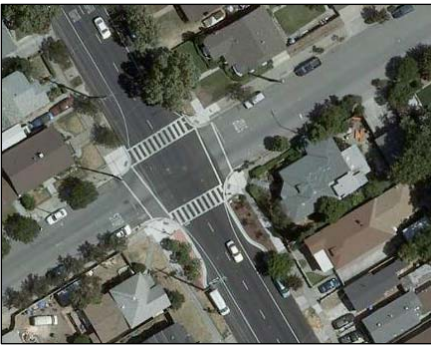
New bulb-outs at Martha Street and South 10 th Street, along with a lane reduction on South 10 th Street, have improved pedestrian safety. Image courtesy of Google Earth, 2008.
