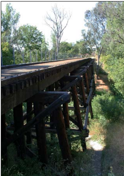
Location of potential second trailhead at Keyes Street and Senter Street (top image) and existing rail bridge over Coyote Creek (lower image).
